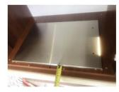
Sit the Base (part 3) on the cabinet bottom with the centre notch at the front. Place it in 20mm from the front edge. Align the centre notch and the centre line marked to locate the base. Ensure the base front edge is parallel with the front.
