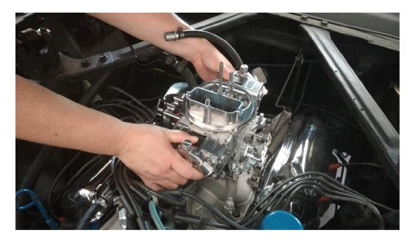
10. Continue installation of the carburetor as is specified by its manufacturer, including reconnecting all vacuum lines, linkages and PCV line as needed.
