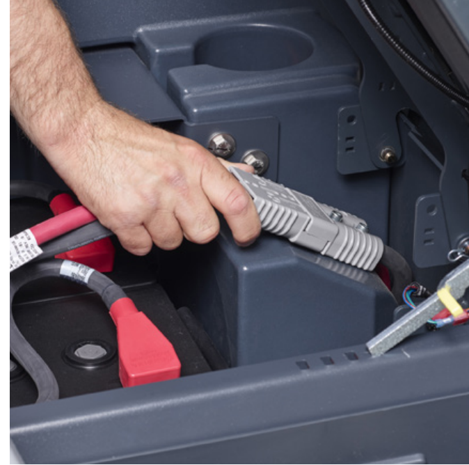
3. Verify the battery cables are properly connected.
