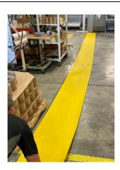
Once in place, apply pressure to adhere the small section to the floor. Flip material along adhered edge. Have two people hold the material in this position.
