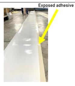
5. \*\* 3 or more people are recommended for step 5 thru 8\*\* Careful not to touch the exposed adhesive to itself, flip the marking over so the exposed adhesive is along the reference line. Adjust the position of the marking as needed to align with the reference and remove any kinks or raised areas before applying pressure the exposed adhesive.
