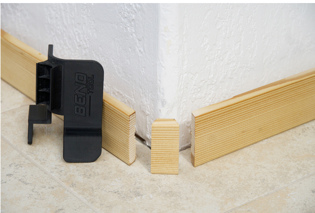
Fig. 2 - Cut and Dry Fit
