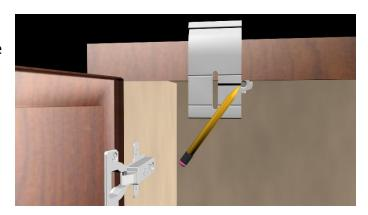
b. Take the bracket that you just marked and position it horizontally on the rear of a wall cabinet with the alignment leg resting on the side of the cabinet. Set the marked bracket about an inch down from the top of the cabinet and use the far edge of the bracket as a guide to draw a vertical line on the back of the cabinet. Repeat at the other end of the cabinet.
