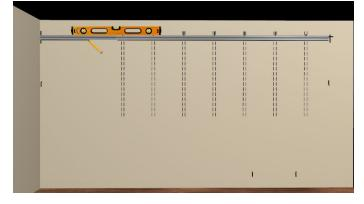
f. Before installing the rest of the black oxide 10 x 2" washer head screws, check the distance from the wall rail(s) ends to the closest wall stud at each end.
