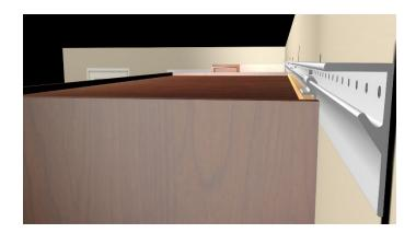
b. The location of the corner cabinet brackets at A will allow for the alignment of the adjacent cabinets on the walls in either direction. Once the corner cabinet is in place you can check the clearance between the cabinet and rail throughout the corner. If the walls are square, you can add other brackets at location B as in the diagram below. If the walls are out of square, you may only be able to attach
