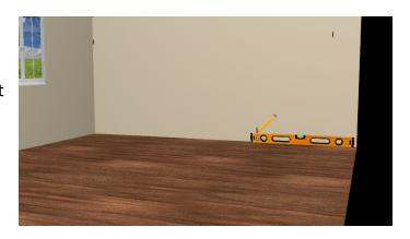
c. At the marked high spot just located, measure up the wall and make a short horizontal mark 13/16" above the height where you want the top of your wall cabinets to be located. This horizontal line marks the EazyHang wall rail mounting hole height.
