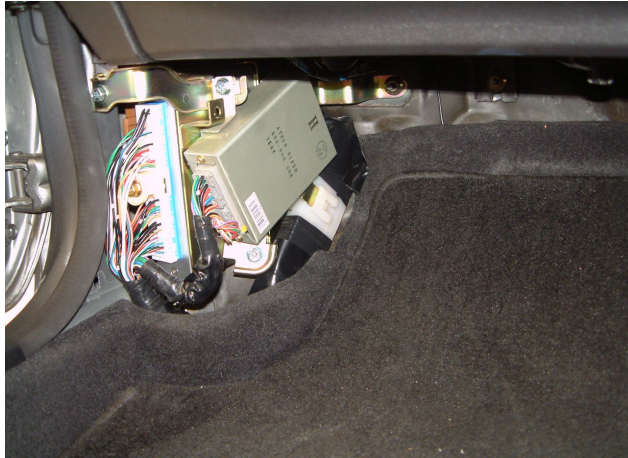
Figure 4 – Haltech ECU Installed
