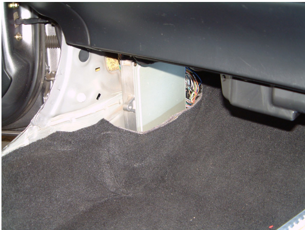
Figure 1 – Passenger side kick panel showing ECU location
