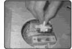
4.put the finished basket in to the origina place, finally close the wood door of fuse.
