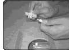
3.take fuse out , the push in a new fuse
