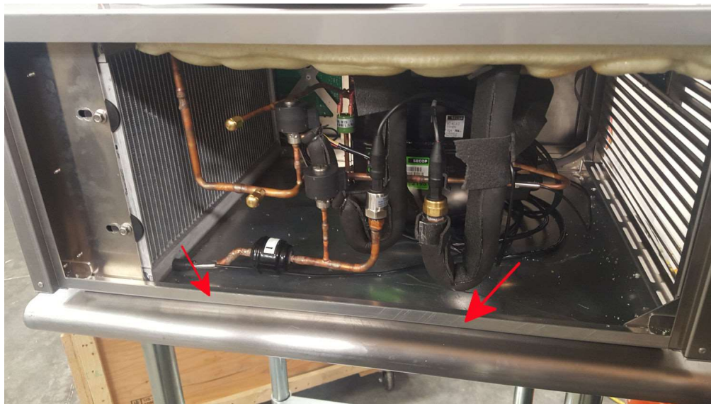
Figure 11: Left panel removal for condenser cleaning
