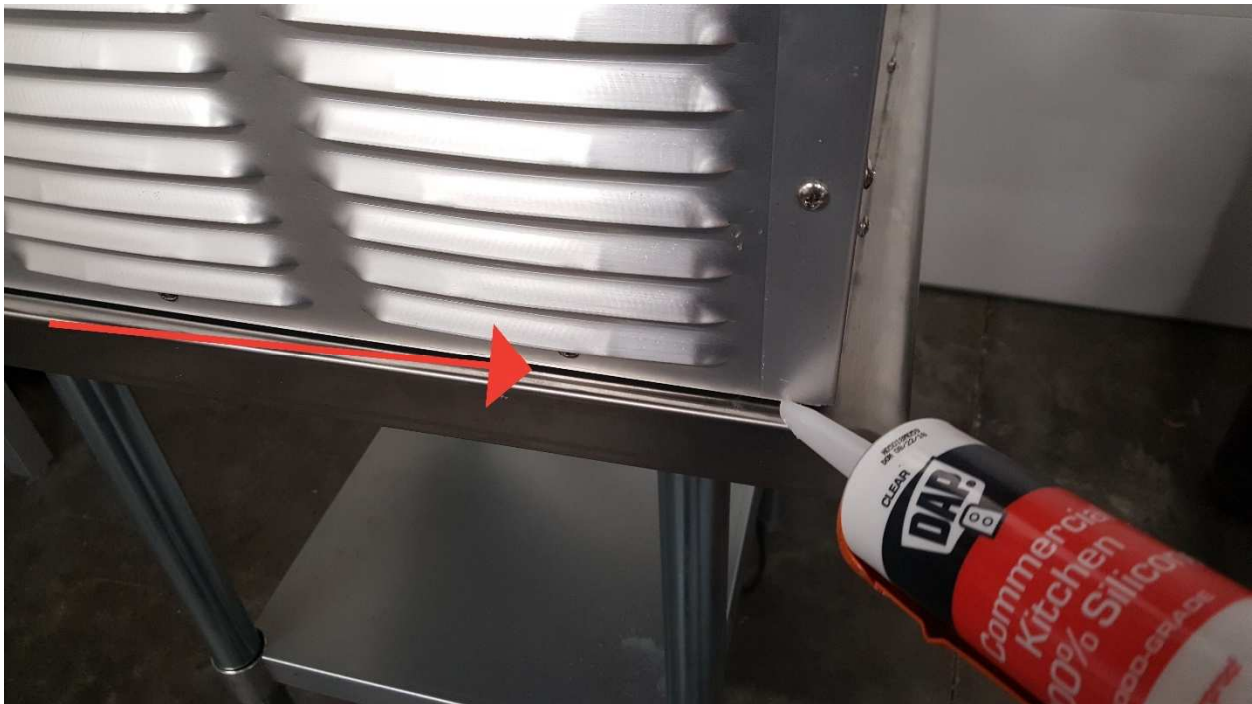
Figure 2: Sealing your unit to the counter or table
