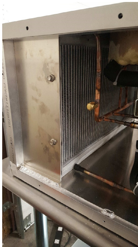
Figure 11: Left panel removal for condenser cleaning
