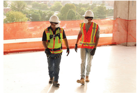
On-site training at your location
