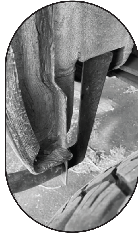
VIEW OF SUPPORT FROM INSIDE WHEEL WELL
