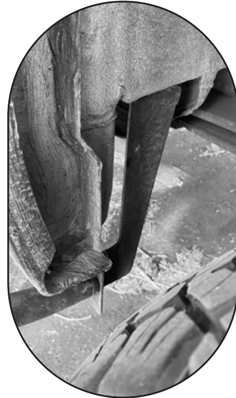
VIEW OF SUPPORT FROM INSIDE WHEEL WELL
