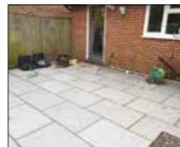
Ensure you have prepared a level concrete base or a properly fitted existing patio or decking with access to a drain.
