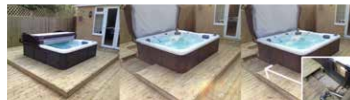
Ensure part of your decking can be removed in order to gain access for future repair or servicing
