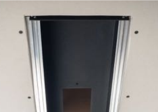
1. D Bay before finishing work
