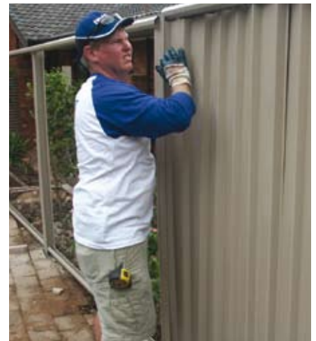
Lift top rail and rotate until infill sheet slides into receiver channel. Tap top rail down into position.
