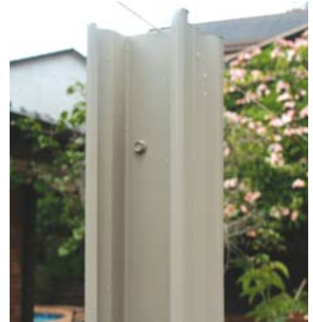
Use stringline to set post heights
