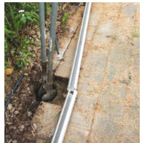
Lay the rails along the string line to determine positions of posts.
