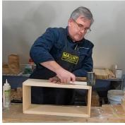
3. Tap the corners together in each direction with a rubber mallet or a hammer with a block of wood to prevent denting the joints.
