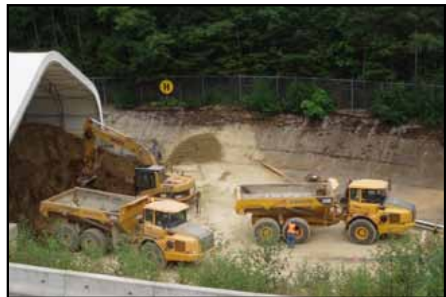
Storing the metal sludge before transport to the Jane Basin pit
