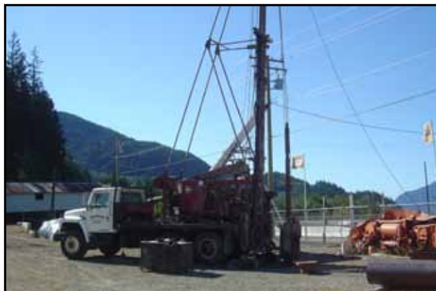
Drilling groundwater pumping wells at the Museum
