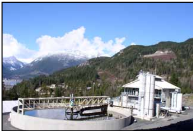
EPCOR Britannia Mine Water Treatment Plant
