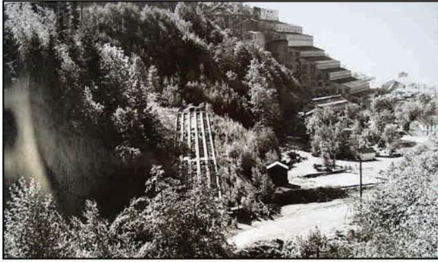
The Beach launders, constructed in the 1950s, were part of the initial water treatment process put in place.
