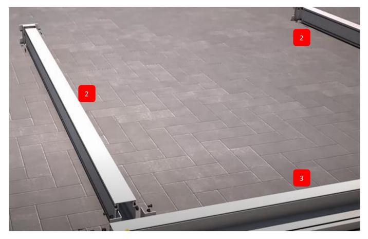
The assembly of Gutter Profile(3) and Pole Profile(2) is recommended on the ground.
