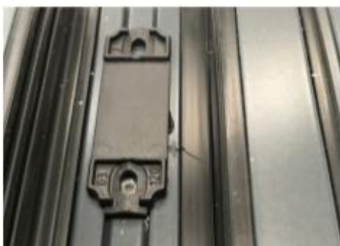
Remove the lock keep and place shaped packer
