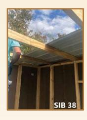
**1.** Hang Right Rear Corner piece First. Leave a 5-inch overhang in the rear. Match even to edge of Rafters. Run screws into rafters.
