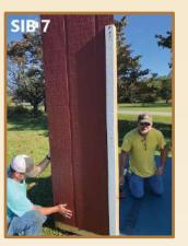
**6.** Attach A3 wall to Left Front corner floor, marked A3 on picture SIB 51.
