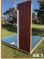
**1.** Attach A1 wall to Right Front corner floor, marked A1 on Picture SIB 51.
