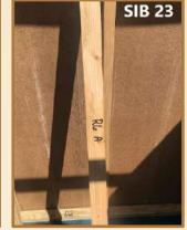
**4.** Hang R6-A rafter by screwing it on top of the left back Wall. Make sure the over hang is the same as other rafters.
