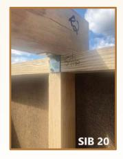
2. Hang R2 Rafter at marked location. Use metal bracket. Over hang should be even on each side.
