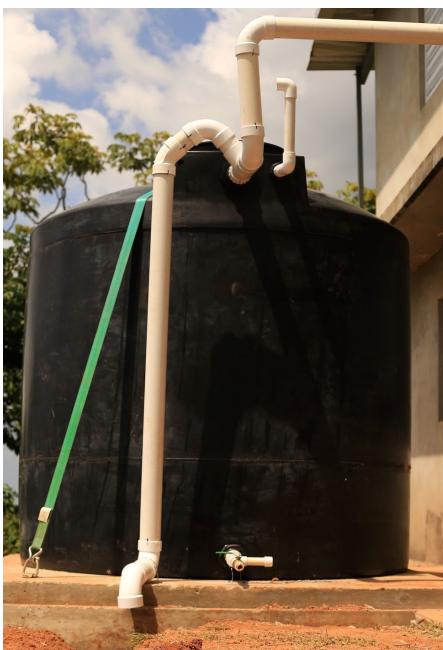
Above Left: The new installed 1,500 gallon cistern harvesting rainwater from the roof of the church. Above Right: Introductory rainwater harvesting & water filtration workshop offered at the church.
