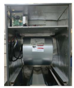
2.) Remove the air duct sealing plate by removing the 4 retaining screws.
