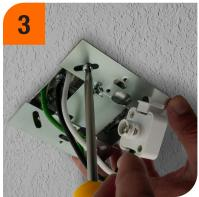
Fasten the mounting plate to the electrical box using the provided screws.
