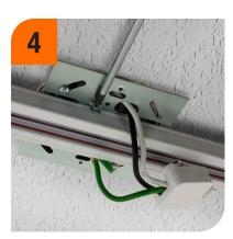
Attach the track channel to the mounting plate using the two screws on the sides.
