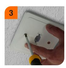
• Screw the canopy to the mounting plate using the provided screws to cover the wires.
