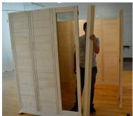
**STEP 13** - Install the (2) 45° corner posts to the narrow wall elements (one wood, the other glass) that frame the door opening. Once the corner post is in place you can nudge it into place with a rubber mallet.
