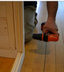
**STEP 7** - Place another 90° corner post to the end element and secure with 6x20 screws.
