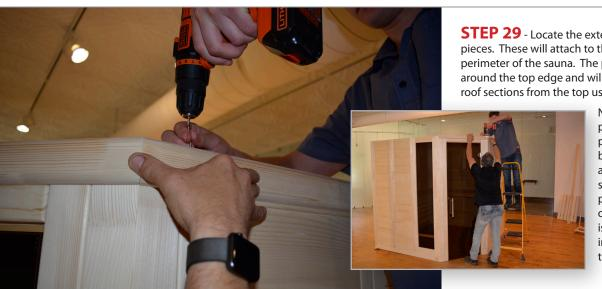
**STEP 29** - Locate the exterior roof trim pieces. These will attach to the exterior top perimeter of the sauna. The pieces create an "L" around the top edge and will be screwed to the roof sections from the top using 3.5x40 screws.
