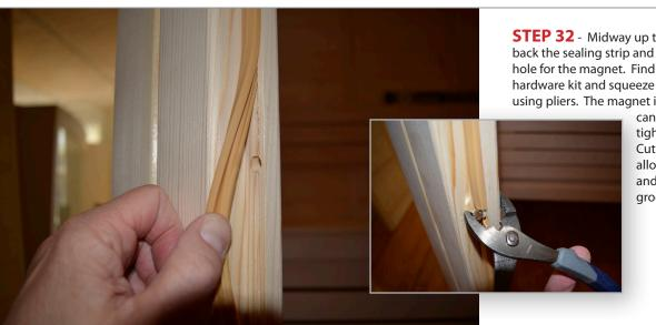
**STEP 32** - Midway up the doorframe peel back the sealing strip and find the pre-drilled hole for the magnet. Find the magnet in the hardware kit and squeeze it into the hole using pliers. The magnet is adjustable and
