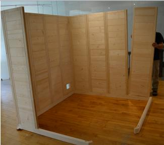
**STEP 8** - Continue the addition of wide wall elements (W) by adding (4) of the wide wall element sections along the second long rail.
