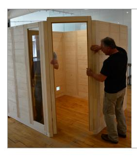
**STEP 16** - In the same way you installed the 45° corner posts, you will now install the doorframe. Raise both sides of the doorframe - you MUST use two people and keep the doorframe level – several inches above the 45° corner posts and then follow the same procedure as in step 13.
