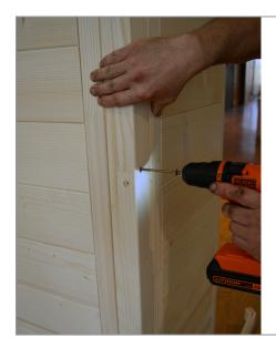
**STEP 5** - Using a cordless drill with the appropriately sized bit (included) use 6x20 screws and secure the 90° corner post to the short and wide element.
