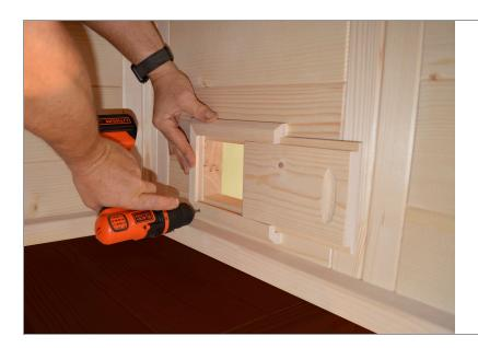
**STEP 28** - Locate the vent cover and position over the wall opening. Attach with (40) 3.5x40 screws.
