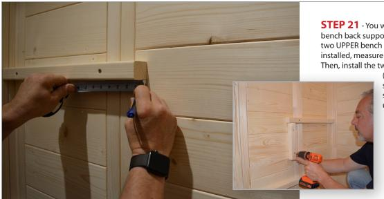
**STEP 21** - You will now install the lower bench back supports. From the front of the two UPPER bench supports that you just installed, measure <sup>3</sup>/<sub>4</sub>" back and make a mark. Then, install the two lower backrest supports
