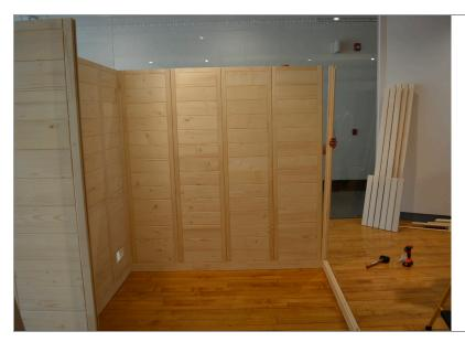
**STEP 9** - Add the third 90° corner post and secure with 6x20 screws as with the other corners posts.
