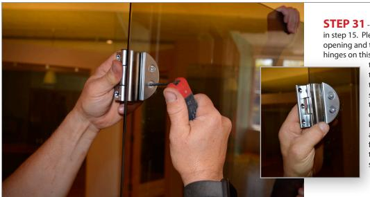
**STEP 31** - Find the board you set aside in step 15. Please it on the floor of the door opening and the place the glass door with hinges on this board. (This allows you to install
