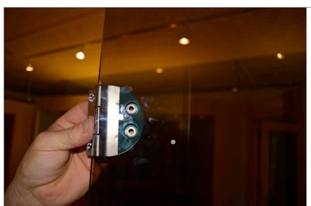
**STEP 30** - Install the hinges onto the glass door. The hinge consists of the hinge bracket, hole spacers, bracket cleat and hex screws. Be sure the screws are snug before mounting the door.
