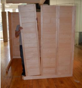
**STEP 10** - Continue to assemble the front short wall by adding (2) of the narrow wall element sections (N) followed by (1) of the narrow wall element sections with the edge clips facing to the door opening.
