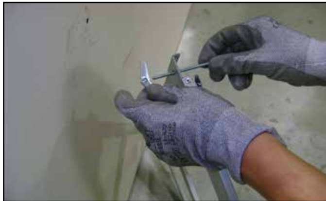
Figure 4.10 Toggle Bolt Installation through Mounting Bracket
