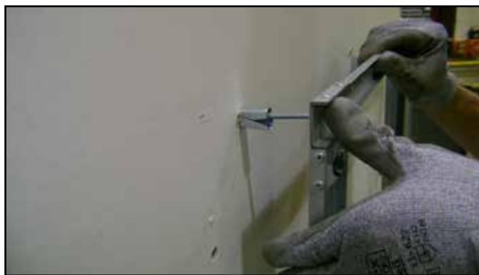
Figure 4.11 Installing Anchors in Hollow Wall
