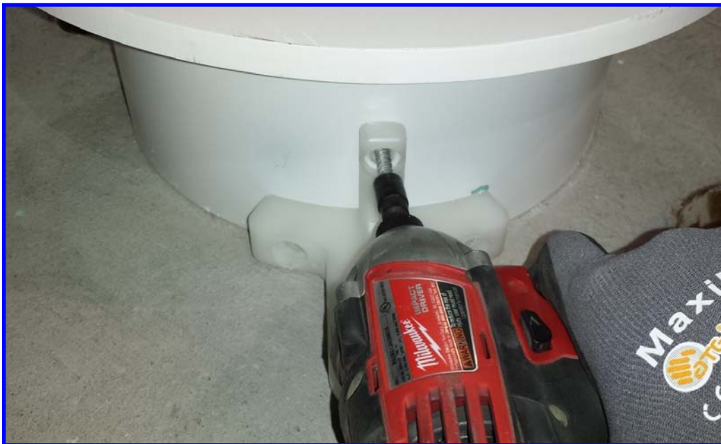
INSTALL THE CONCRETE SCREWS (5/16" DRIVER OR SLOT SCREWDRIVER)
