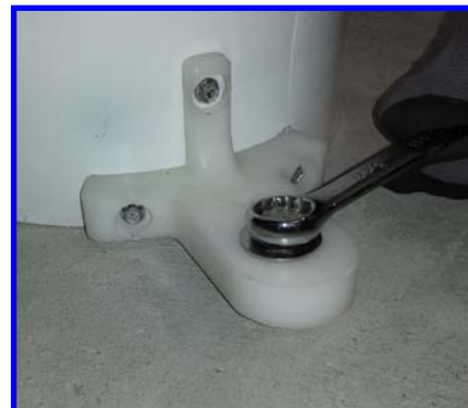
TIGHTEN WITH 3/4" WRENCH TIGHTEN UNTIL BOLT IS FLUSH DO NOT OVERTIGHTEN!
