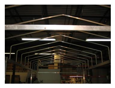
Bolt the canopy top bow support (2 sections) using (2) 1  $\frac{1}{2}$ +x  $\frac{1}{4}$  carriage bolts and (2) nylok nuts. To ensure you have the proper alignment maintain a 24+gap between the pre-drilled holes.
