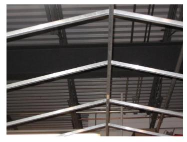
Secure the side top rails in the upright saddle brackets using (4) 3  $\frac{1}{2}$ +x 3/8 hex bolts, (8) flat washers, and (4) nylok nuts.
