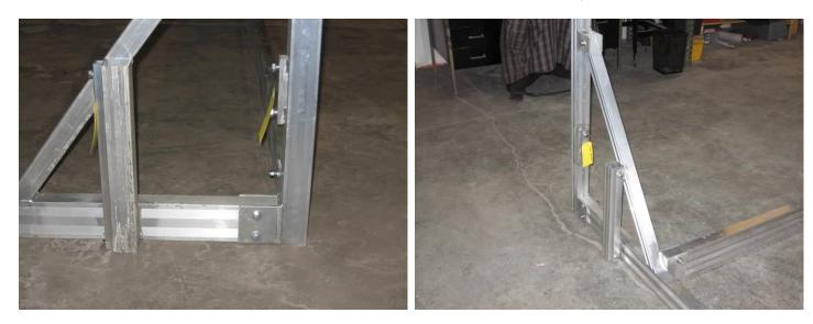
Secure the right side with (10) 3  $\frac{1}{2}$ +x 3/8 hex bolts, (20) flat washers, and (10) nylok nuts.
