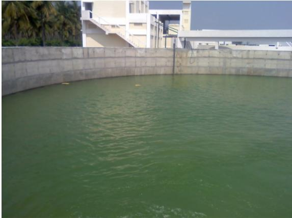
Equalization Tank: 36m $\Phi$  x 4m deep
