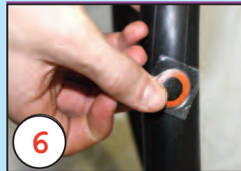
6. Stick the repair patch on
