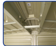
Strong Steel Roof Truss Carries 20 lbs/sqft Snow Load
