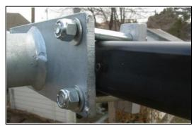
Place longitudinal tubes on top of crosspieces and bolt with square washers on top and bottom.
