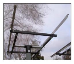
When fastening panels to rails, place first panel at end of rails marked "Top" and work down until all panels are in place with bolts finger tight. Cross measure array for square, check to see that all spaces between panels are equal (at least ¼"), **then tighten all bolts with wrench.**
