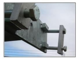
Place Tee assembly on top of post. Tighten both set bolts and the four bolts on the top of the "Tee". Align center tube east and west and tighten two square head set bolts to post. Finger tighten the aluminum flat bar and straighten  $\frac{1}{2}$ " bolts onto "Tee" endplates on the center tube. Slide crosspieces into the flat bar arrangement. Make sure to locate the lugs on
