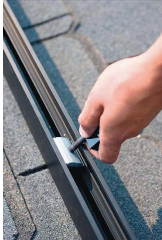
Snap module clamp assemblies into rail
