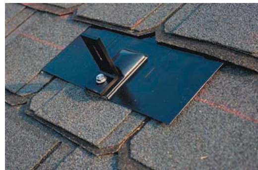
Installed L-foot assembly
