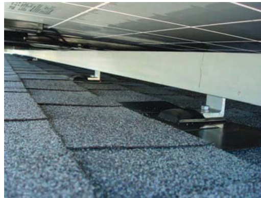
Check under the array for dangling wires
