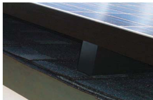
Rubber end cap installed
