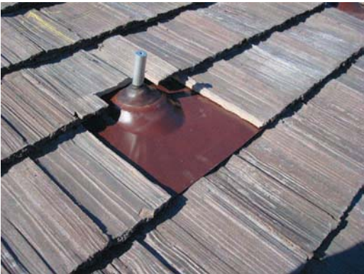
Standoff installation using Oatey flashing
