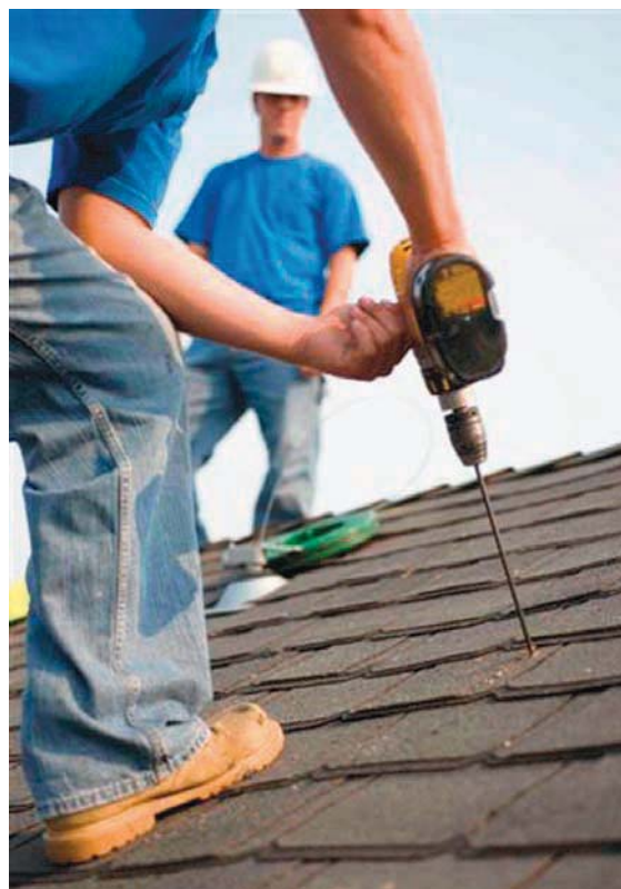
Drill pilot holes
