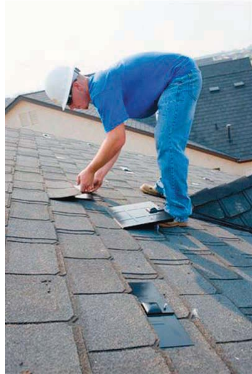
Install flashing
