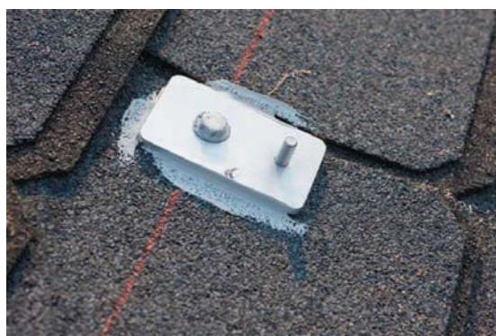
Apply sealant and secure base to rafter
