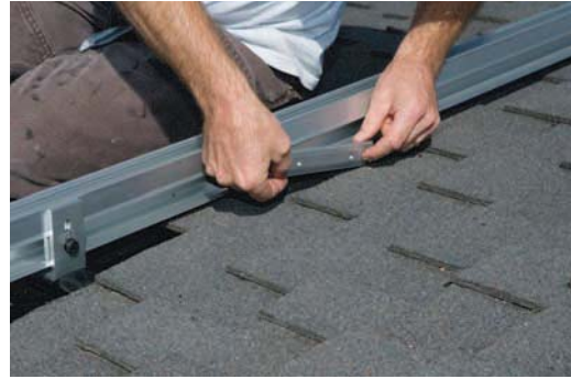
Snap in channel nut
