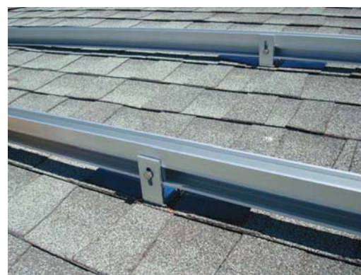
Standard rail mounting configuration
