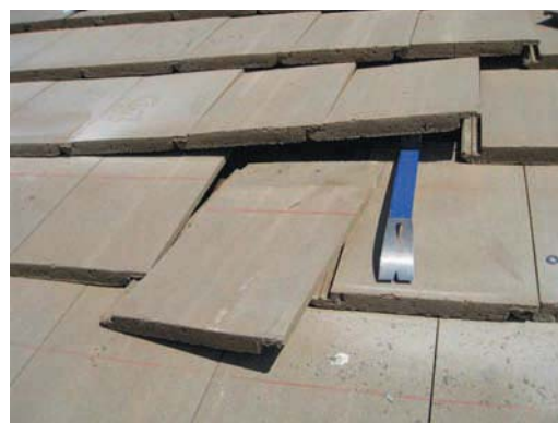
Remove roofing material to expose roof underlayment
