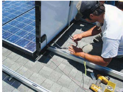
Connect wiring
