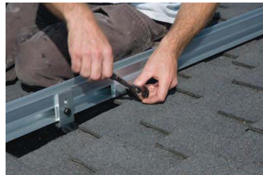
Tighten bolts on splice
