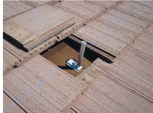
Screw standoff onto base
