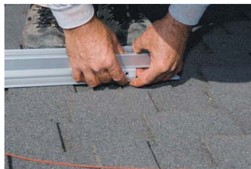
Snap in channel nut
