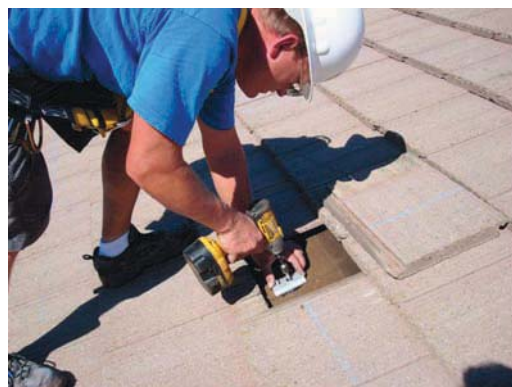
Secure standoff base to rafter
