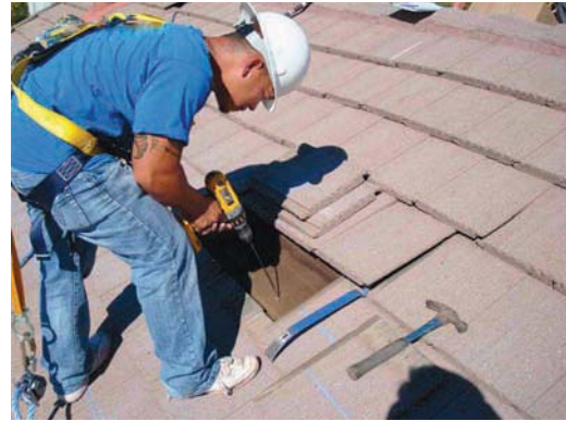
Drill pilot holes
