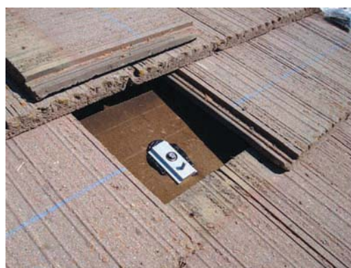
Typical standoff base installation
