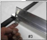
Then roll the rails over so the bolts slip into the holes on the panel frame. Place the flange nut on your finger with the flange UP and thread onto the bolt from underneath as shown in Photo #3. Finger tighten.
