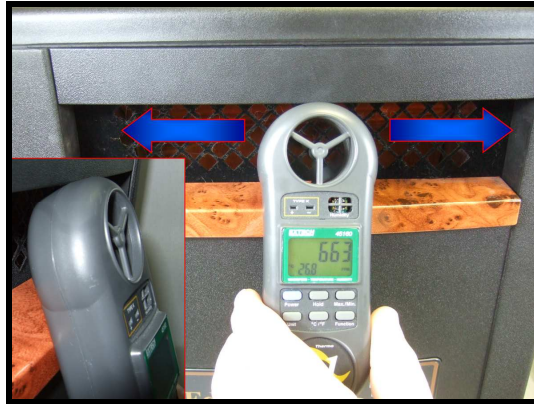
(FIGURE A) AIRFLOW TESTING
