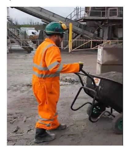
ezTip Safety Handles being used on an oversized laden wheelbarrow.
