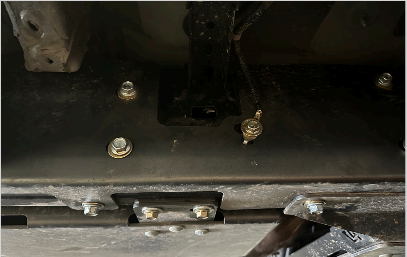
Figure 3: Ground wire reattached
