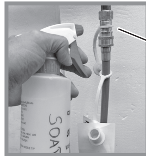
QUICK-DISCONNECT COUPLING CONNECTION AT GAS SUPPLY
