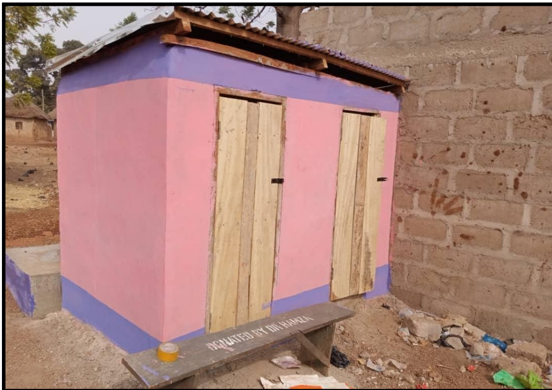
Example of Pit Latrine Constructed at Shea Butter Processing Center
