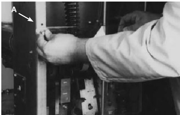
Figure 33. Attaching CloSure test tool at hole "A".
