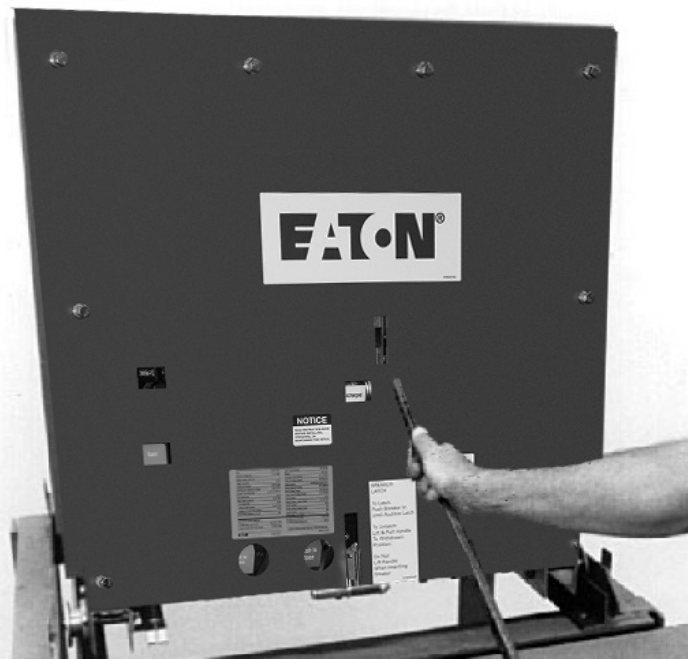
Figure 8. Type VCP-W circuit breaker manual charging handle in use.
