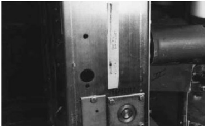
Figure 41. Place the tape on the right side panel of the breaker.
