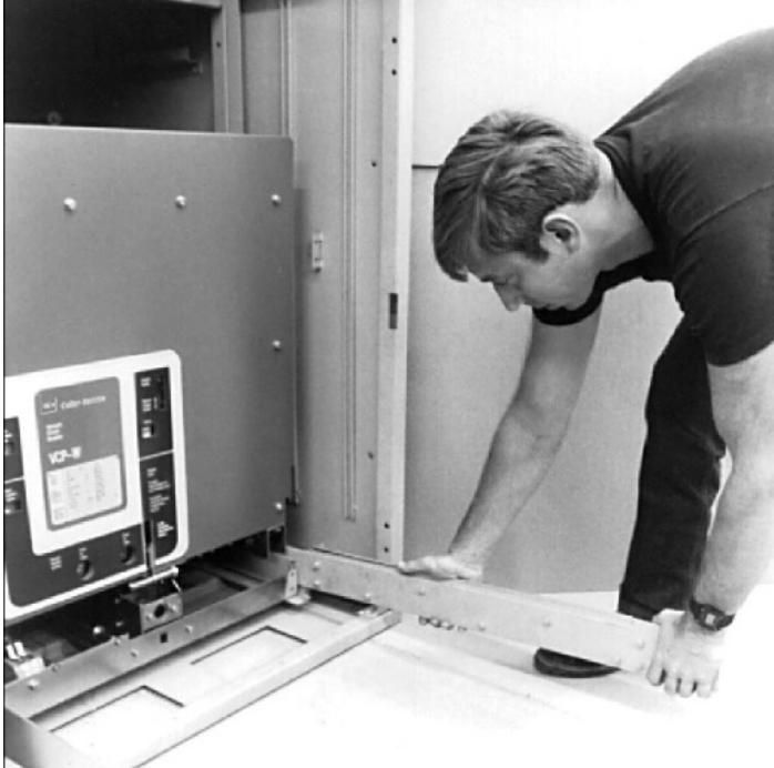
Figure 14. Engaging extension rails in a lower circuit breaker compartment.
