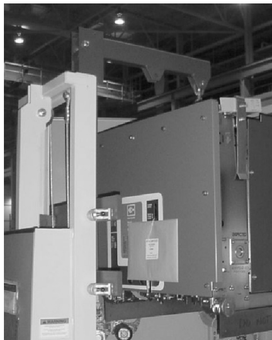
Figure 10. Lifting and setting the breaker in the housing.
