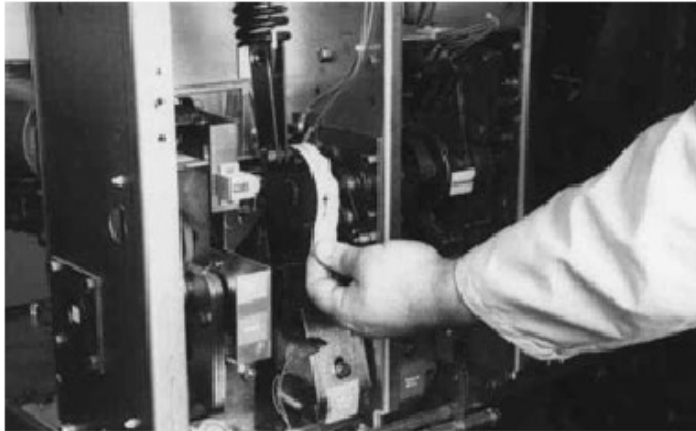
Figure 40. Remove marked masking tape from the cam.
