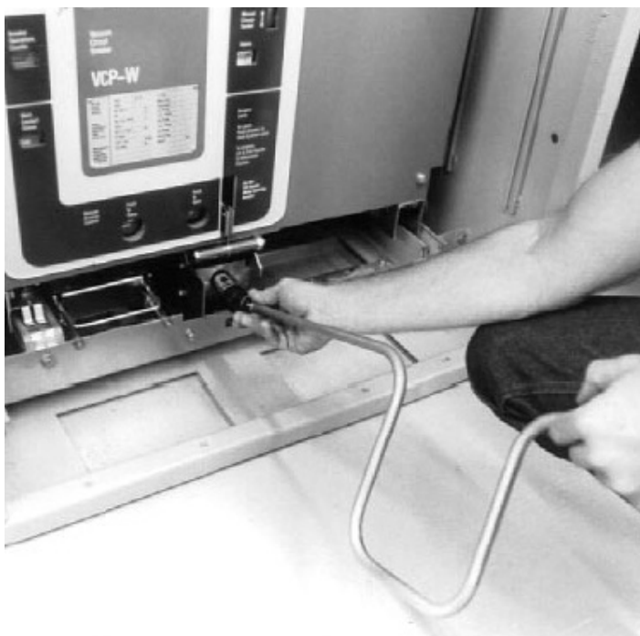
Figure 17. Engaging levering-in crank.
