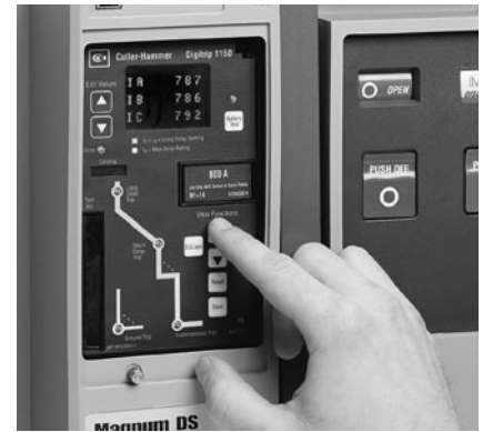
Digitrip RMS 1150 Programmable Trip Unit
