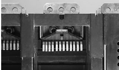
Visual contact wear indicator shows when contact replacement is necessary.
