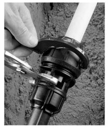
**4. Nut Tightening** Tighten nut firmly with a wrench. Nut will not butt against the body flange when the pipe size is at the top end of the fitting tolerance.
