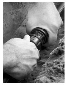
**4. Nut Tightening** The nut should be tightened by hand and then firmly with a wrench. Tighten the nut all the way to the flange on the body of the fitting.
