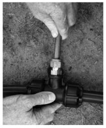
**3. Pipe insertion** Insert the pipe and push it past the olive.
