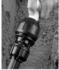
**3. Pipe Insertion** Insert the pipe to the correct depth. Always ensure the nut is backed off and 3 threads are showing. Pipes at the top end of the fitting tolerancemay require 5 threads showing.
