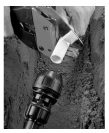
I. Cut Pipe to Length The fitting is pre-assembled and ready to use. Cut pipe square and to length using the flange on the central body as a guide. Ensure the end of connecting pipe is undamaged and clean.
