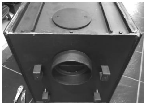
The flue and blanking plate are then swapped over. Be careful to ensure good air-tight seals are maintained on the new attachments – use fire cement if necessary
