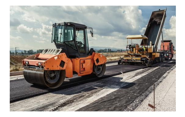
"PG-5000" is designed to provide better release for all high asphalt content mixes. PG-5000 is a stable blend of biodegradable soy oil, along with emulsifiers. When mixed with water, the resultant mixture leaves an extremely slippery film on the surfaces, which prevents the hot asphalt from adhering tightly to the metallic surfaces.
