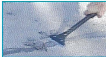
3. Excess material can be shaved after 10-15 min.
