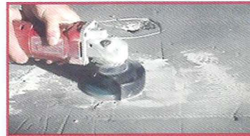
8. Ready to grind smooth in just 20 minutes
