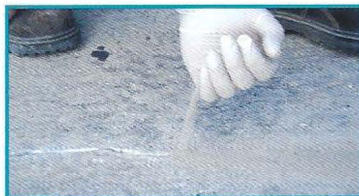
1. Sand can be added to For use as filler
