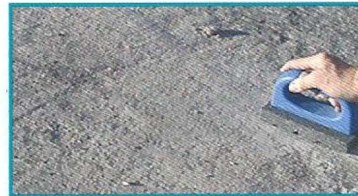
4. Sand if desired after fully cured
