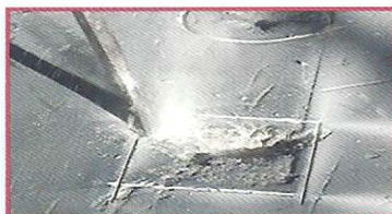
2. Remove feathered edges with chipping hammer
