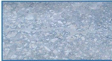
6. Ready for traffic in 20 min.
