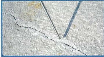
2. Clean with compressed air
