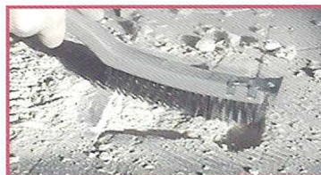
3. Remove debris. Brush, clean with comp. air
