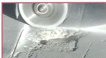
1. Saw cut around outer edges of spall
