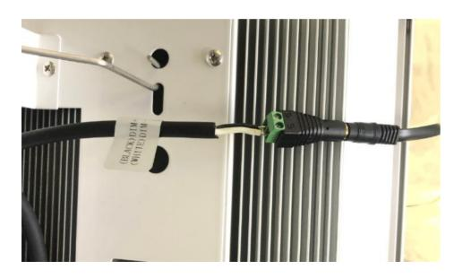
Black Wire of Fixture (DIM +) to (+) of Terminal Block
