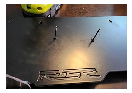
Match the airfoil with the existing holes and with your rivet gun, rivet them into place like in the picture above. Repeat this process for the other 3 airfoils.
