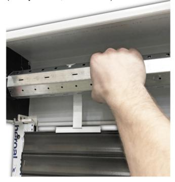
(7.7) Using the tape pull/wind mechanism, retract curtain into the hood assembly. Guide slowly to avoid damage.
